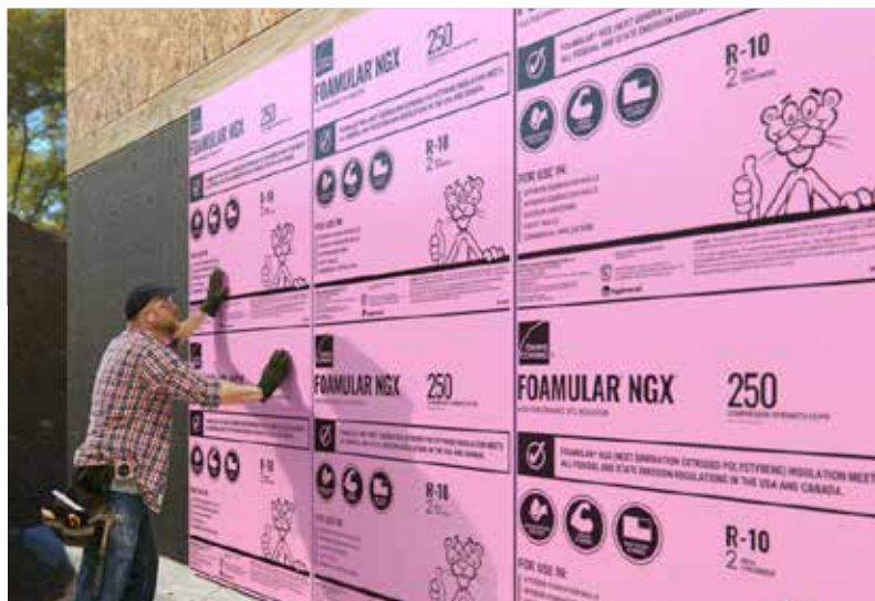
Photo: FOAMULAR® NGX™ insulation being installed.
